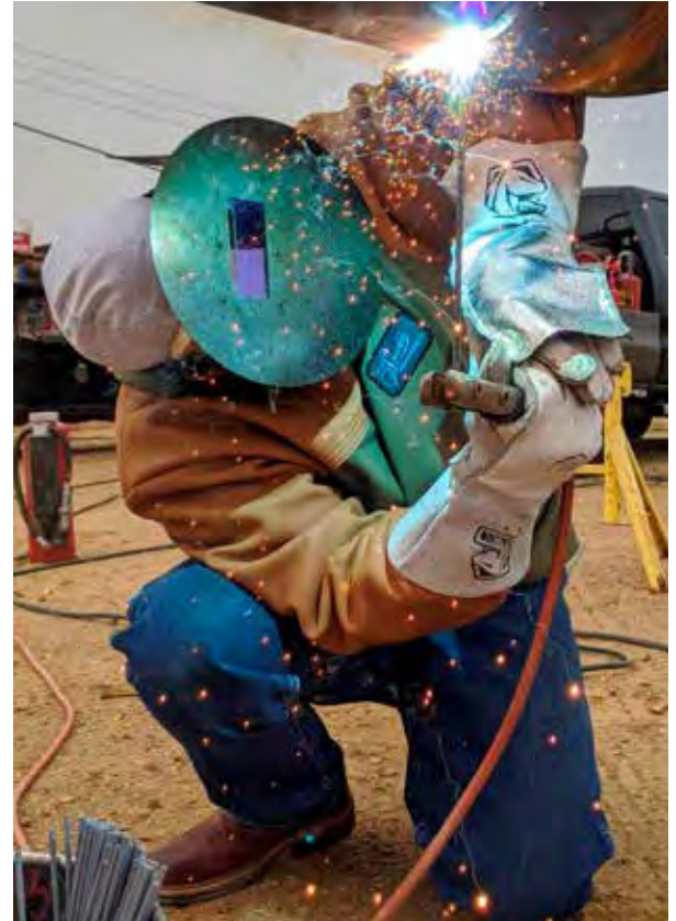
Pipeline welder photo on cover and page 2 credit to: Ryan Kirkland @kirklandwelding
